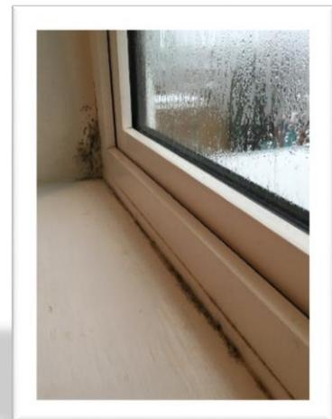
*A typical example of surface condensation. Mould growth can be seen in the corner.*
